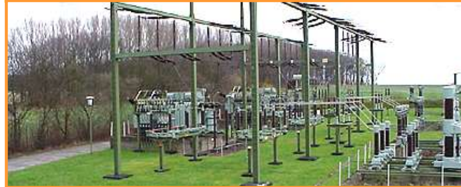
Air-Insulated Substations
