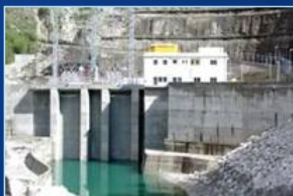
HPP MESSOCHORA, 2 x 90 MVA GREECE
