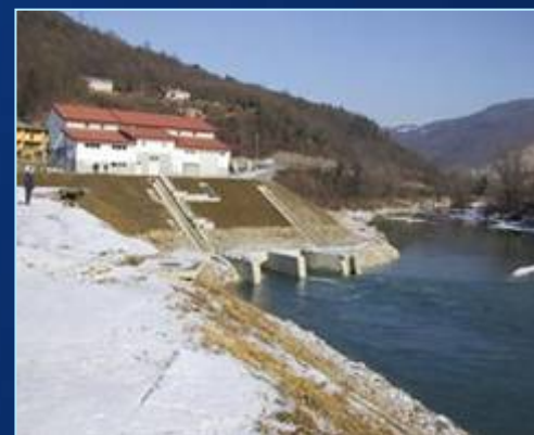
HPP PLAVE, 1 x 23 MVA SLOVENIA
