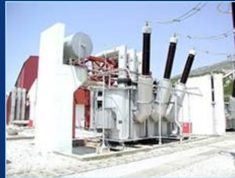
SS ERNESTINOVO AUTOTRANSFORMATOR 420 kV/ 300 MVA CROATIA
