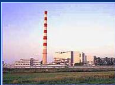
CCPP NOVI SAD, 1 x 194 MVA SCG
