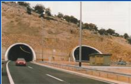
TUNNELS Electrical equipment CROATIA
