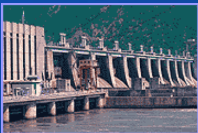
HPP ĐERDAP, 3 x 190 MVA, SCG
